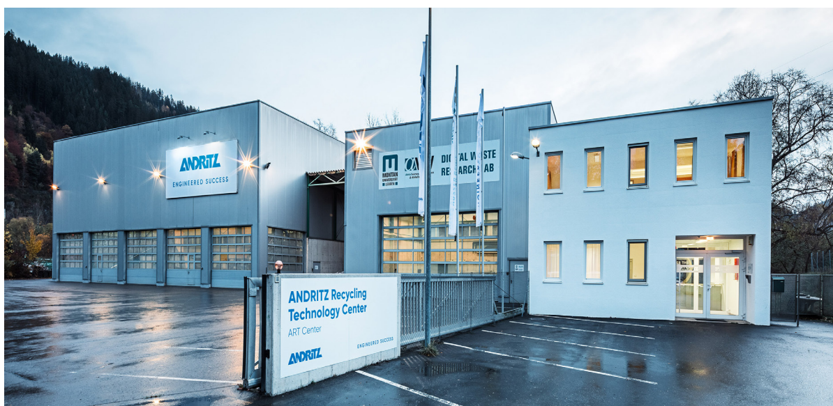
Abb. 1: Standort des DIGITAL Waste Research LAB in St. Michael, ANDRITZ Recycling Technology Center (ART-Center), Quelle: ANDRITZ Recycling
